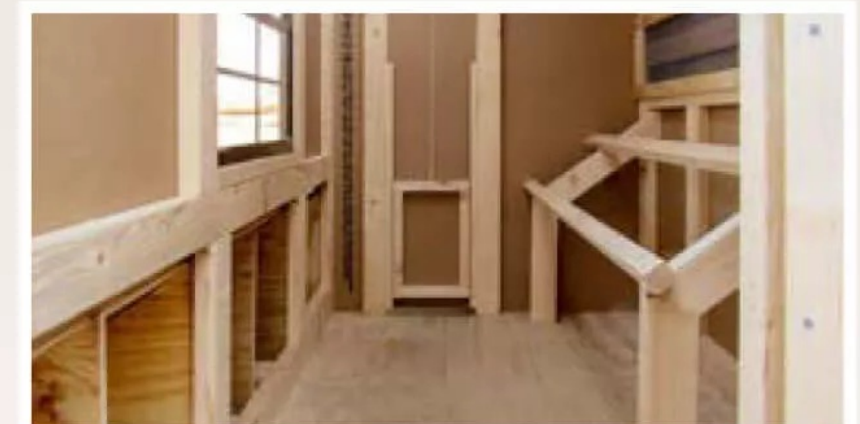
Interior view showing chicken door, vents, roosts, nesting boxes and feeder
